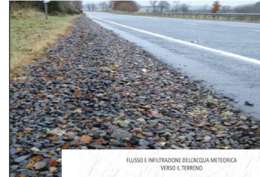
Trincee infiltranti – IT
