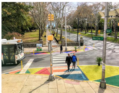
Curb extension design (Street Plans)
